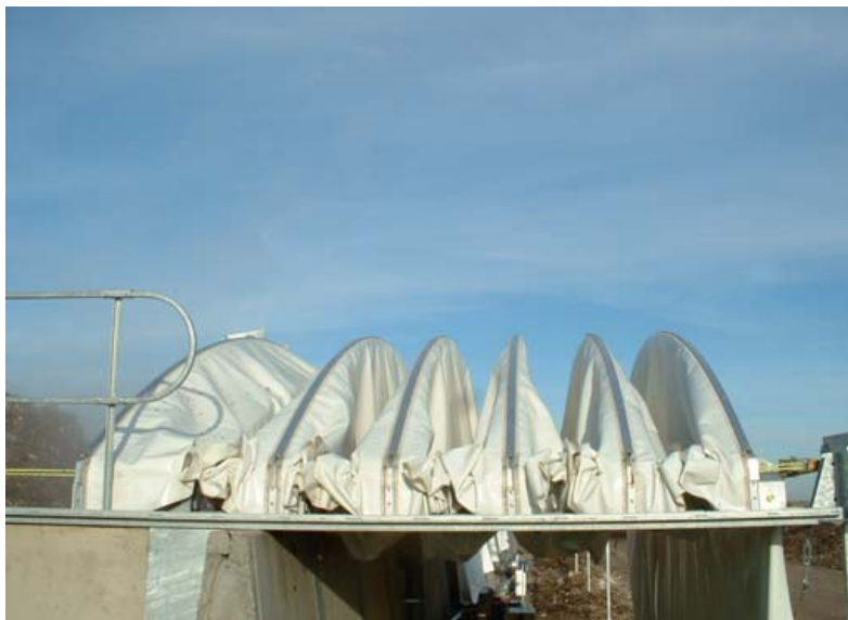
Photograph 5: Roof concertinas to the back wall of the vessel
