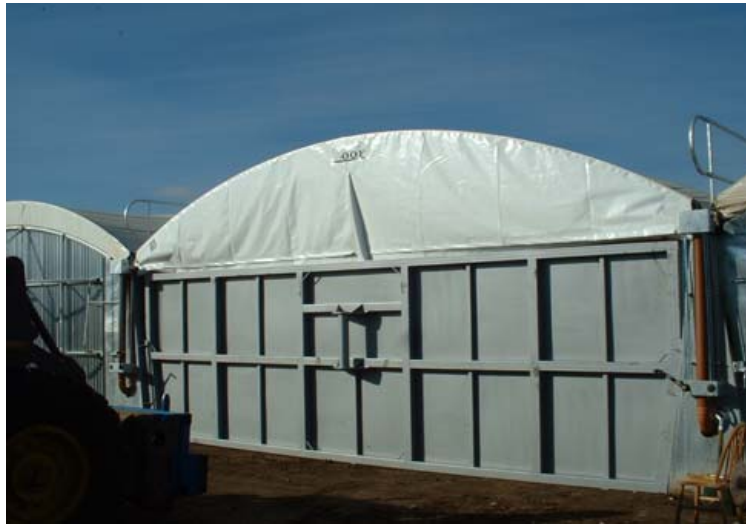
Photograph 10: Door in place, roof brought forwards
