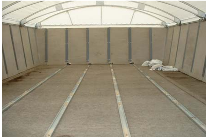
Photograph 7: Air pipes
