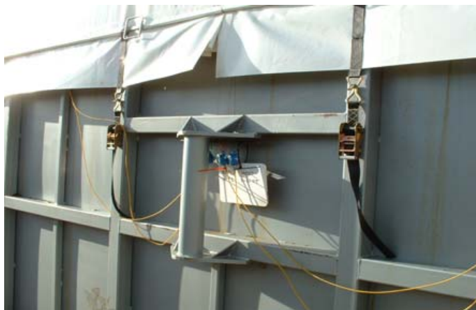
Photograph 12: Roof flaps secured
