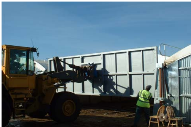
Photograph 11: Door being lowered into position
