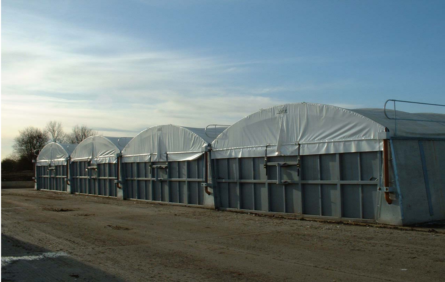
Photograph 13: Front view of four vessels
